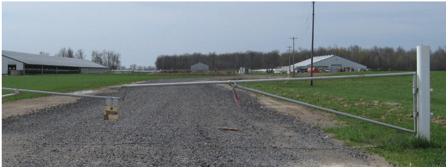
March, 2012 – The former Vreba-Hoff facility #2 south of Hudson on US-127 is locked up.
